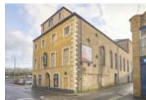
Georgian society: Grand Theatre (1781). Rendered sandstone rubble, slate roof. Main facade has chamfered quoins and is of 3 storeys and 4 bays.
