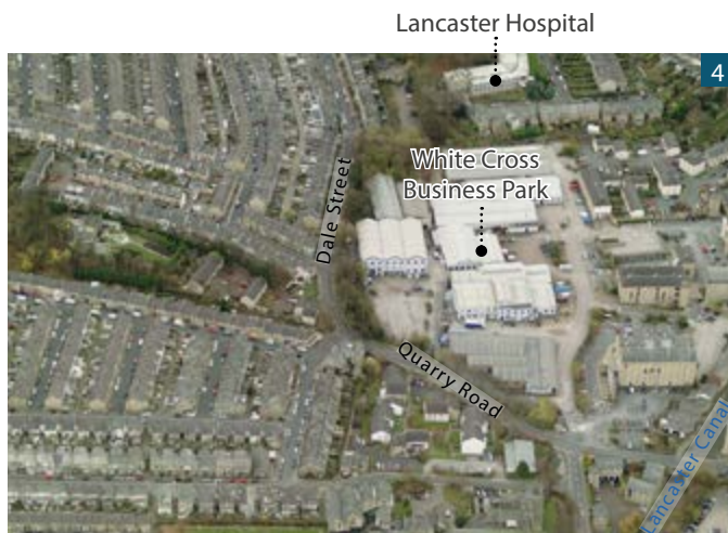
Aerial photo of the south of the site with residential and large retail/light industrial use.
