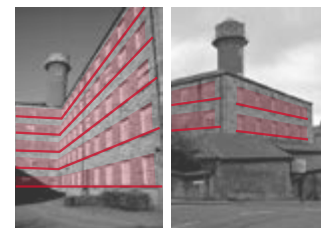
Moor Lane Mill South: Landmark building part of historic mill complex. Simple detailing further emphasises extremely regular horizontal layers.
