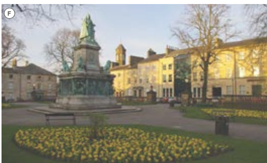
Dalton Square: 1906 redesign. Stone balustrades, simple flag paving, mature trees, grass, Queen Victoria statue central feature. Paving could be improved and statue better maintained.
