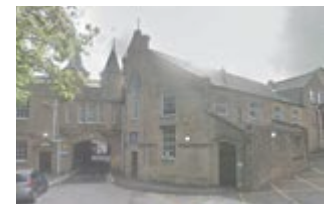
Former Baptist Chapel and White Cross Mill gatehouse: Chapel built in 1872, integrated into the Mill complex in 1894, and new gatehouse built (1899) creating a Mill entrance near Penny Street Bridge.
