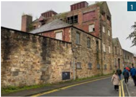
The Brewery building.
