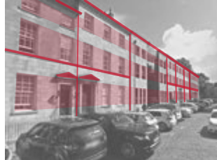
Dalton Square east side: Georgian homes converted to offices, with some recent office infill development. Unified horizontal windowline, vertical bays of 2 or 3.
