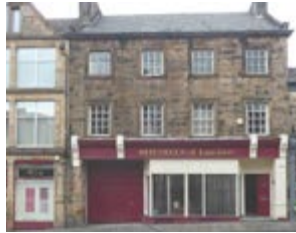
Listed home and shop front, Moor Lane
