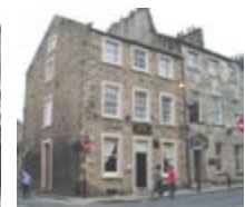
Inns were built to serve travellers between England and Scotland. The Sun Inn, Church Street (1785). Georgian period building of rubble faced sandstone.
