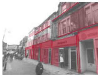
Cheapside: Late 19th century ground floor timber shop fronts form strong horizontal plinth atop of regular vertical glazed bays. Three storey residential buildings (mixed Georgian/ Victorian), two horizontal upper layers.
