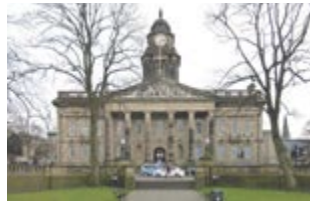
Civic: Town Hall (1909), Grade II* listed city-wide landmark. Edwardian Baroque style, rich carved details. 2 and 3 storeys, pedimented 11 bay entrance elevation. Sandstone ashlar, slate roof.
